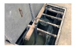
Two SulfiLogger™ sensors were permanently monitoring dissolved H<sub>2</sub>S in the raw sewage at two influents at the wastewater treatment plant in Cassis.
