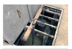
Two SulfiLogger<sup>™</sup> sensors were permanently monitoring dissolved H<sub>2</sub>S in the raw sewage at two influents at the wastewater treatment plant in Cassis.
